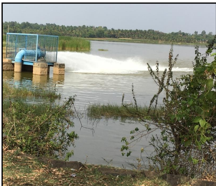
Photo 1: Filling of existing irrigation tanks with water from Shimsha(Iggalur Barrage) at Garkahalli, Harekoppa GP, Channapatna Taluk
